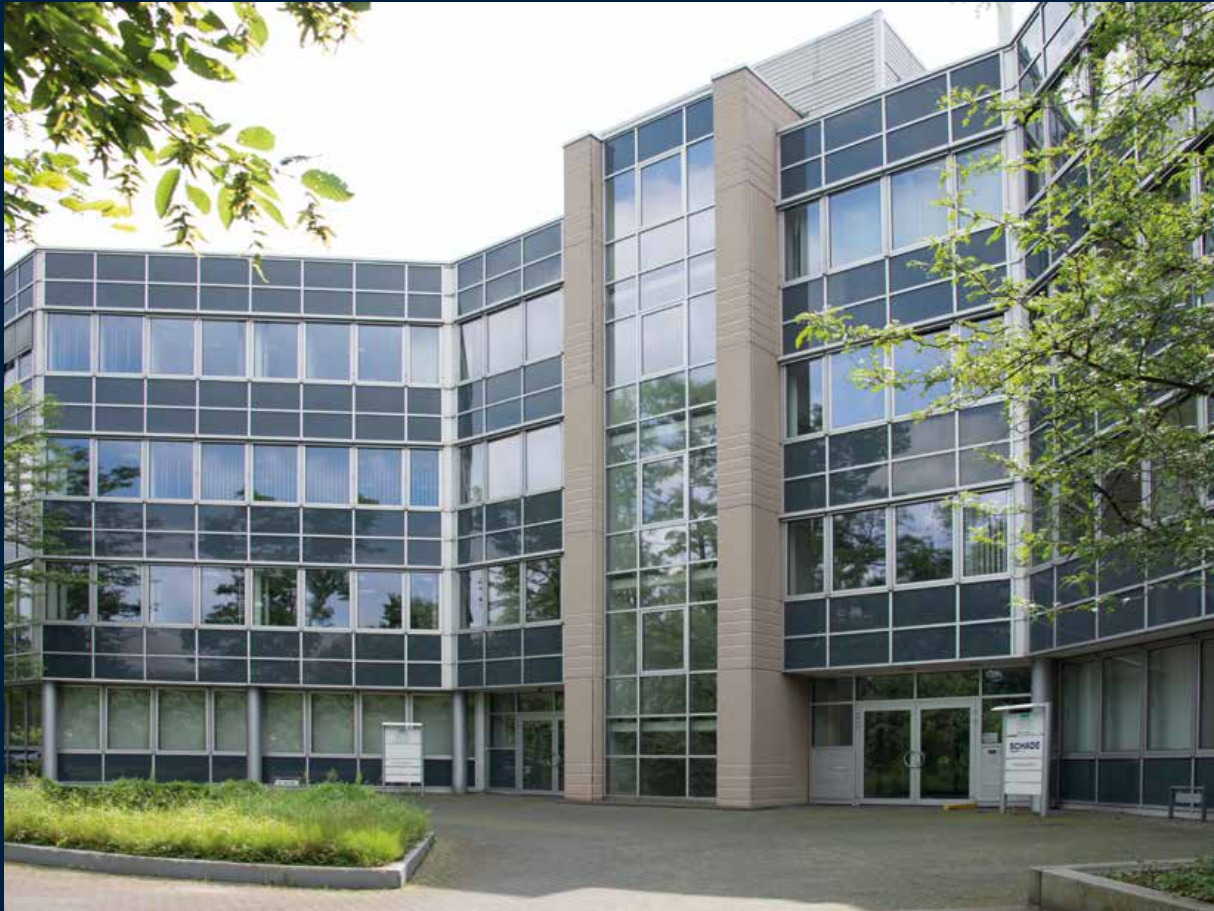
SCHADE Headquarters Gelsenkirchen, Germany
