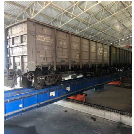
Photo 2: Triple Wagon Traverser/Transborder, operating at 20 cycles (60 wagons) per hour
