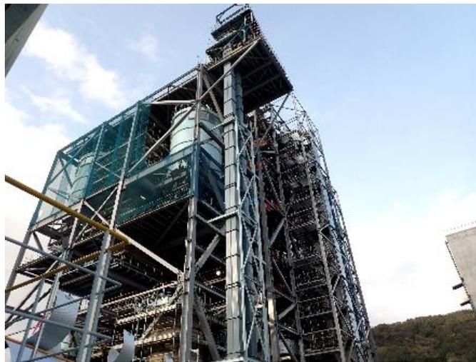
The AUMUND Bucket Elevator with Gravity Discharge type BWZ-S has been in operation in the power plant at Ofunato since autumn 2019 (© AUMUND).
